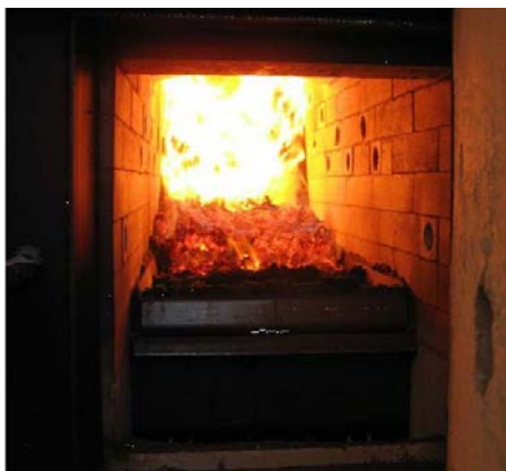
Inside of boiler
