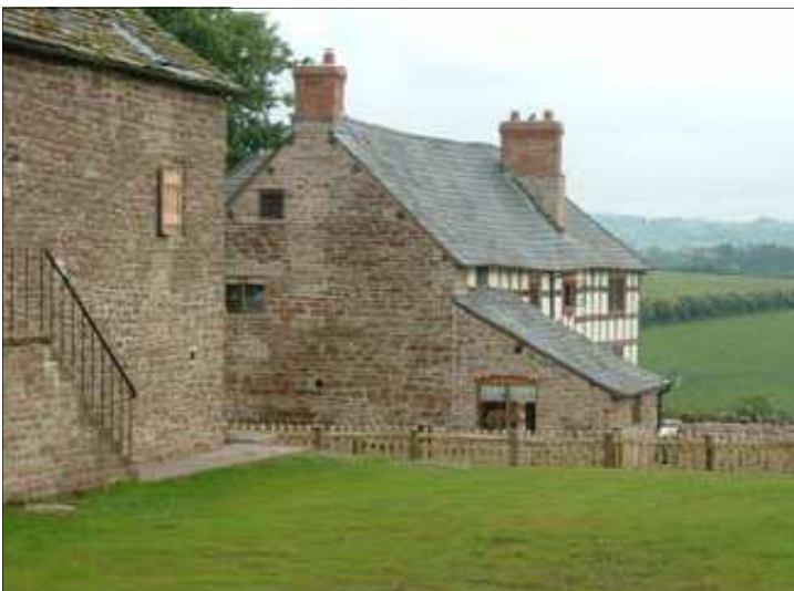
Above; The rear of The Granary and Farmhouse
