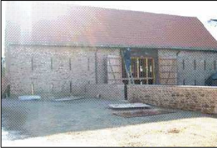
Above; The Great Barn, during restoration
