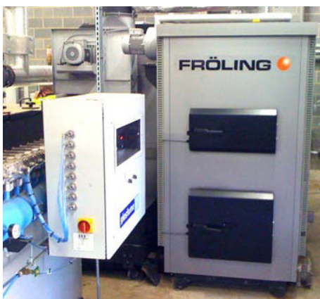
Turbomat boiler and Glosfume Ceramic Filters
