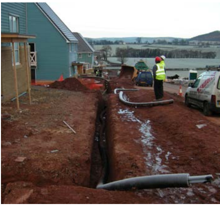
District heat mains being installed
