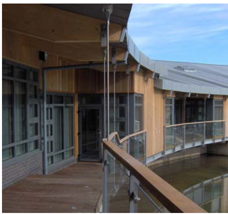
Enclosed glass walkway
