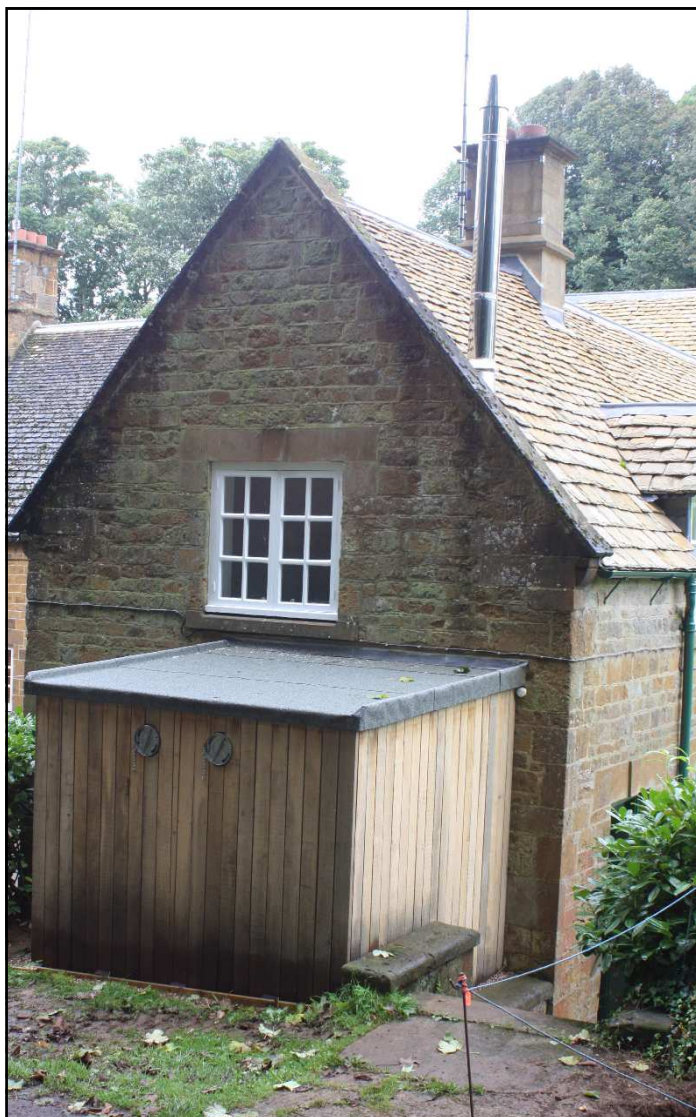
Left - Purpose built pellet store, showing storz 'A' pellet connections.
