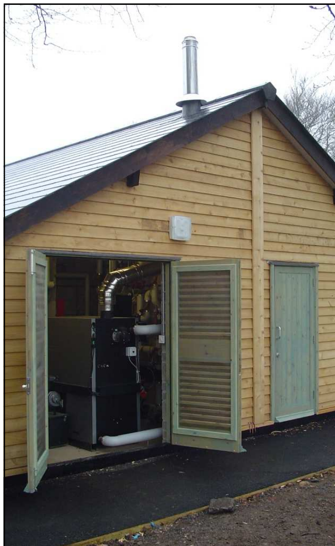
Above; Boiler room and fuel store (right)
