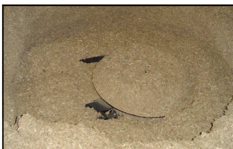
Left; Spring arm outfeeder within the fuel store Below; Aerial shot of the centre.
