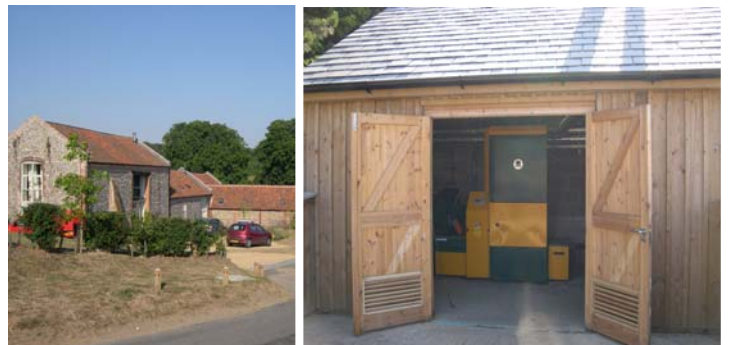
Below: The Lowes , a traditional Norfolk flint and brick farmstead, has been converted into 11 luxury rental properties and an indoor pool which are heated and controlled by a single KWB wood boiler
