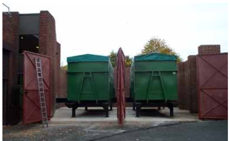
The hook-lift bin fuel delivery system
