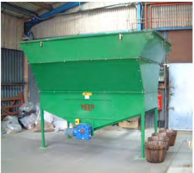
The hopper holds up to 10m 3 of chipped woodfuel
