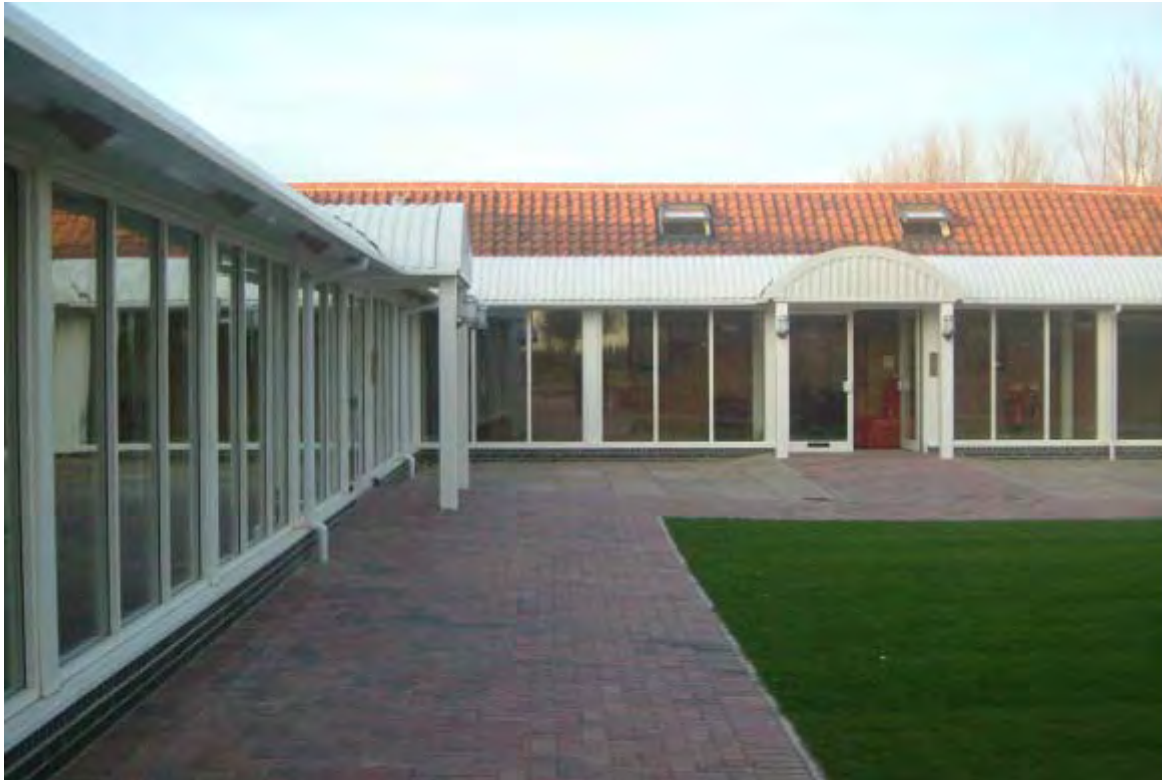
Newly converted office units, all with underfloor heating fed by the woodchip boiler
