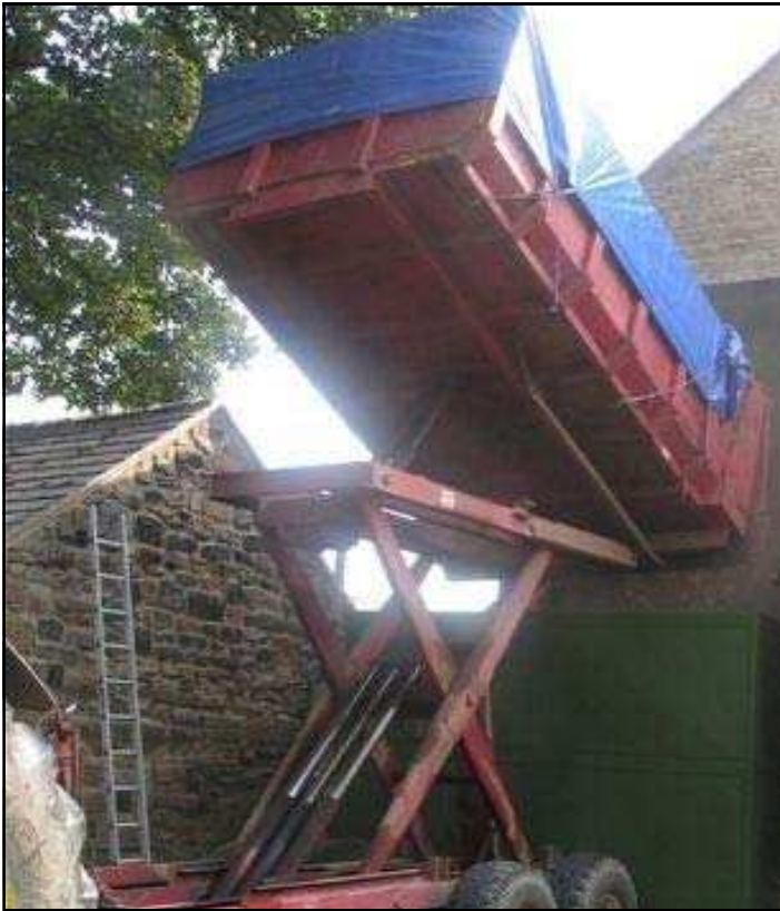
Left; Woodchip delivery Above; Hydraulic hopper lid open for fuel delivery Below; The purpose built boiler house and Econergy designed steel hopper
