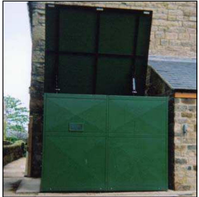
Left; Woodchip delivery Above; Hydraulic hopper lid open for fuel delivery Below; The purpose built boiler house and Econergy designed steel hopper
