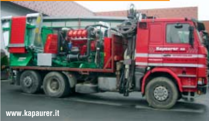
T9 - Scania engine 510 HP, contractor Kapaurer
