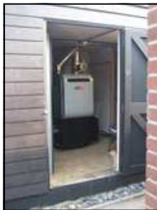
35kW Pellet boiler Village Hall in Suffolk. Ecoexcel
