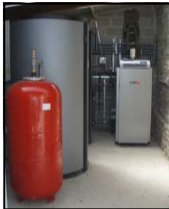
35kW Pellet boiler Village Hall in Suffolk. Ecoexcel
